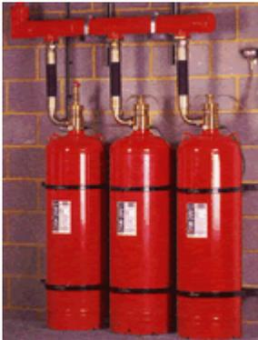
These agents are non-conductive, non-corrosive, and some can safely be discharged in occupied areas. The name "Clean Agents" is commonly used because they leave no residue and cause no collateral damage. For years Halon has been used as the agent of choice, however, it was phased out in commercial applications due to its ozone depletion properties. We will discuss Halon alternatives in the next section. The
