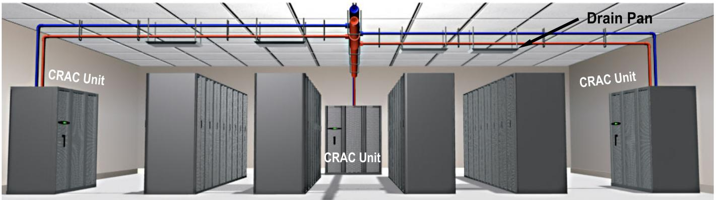
With the valves being located above the ceiling or outside the data center, balancing the cooling system is not easily done. This increases the time required for start-up and balancing of each unit. In case of leakage in an overhead installation, the repair must be performed above the equipment installed on the floor, which increases the potential for water on the floor or worst yet, the equipment.
